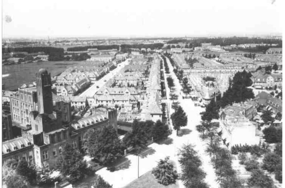
At the left-hand side the Prins Hendrik barracks
